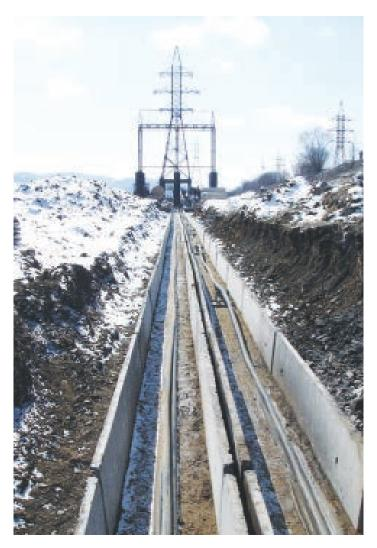
During XLPE 110-220 kV cable laying the bending radius shall be at least 15xD, where D — outside cable diameter. When cables accessories installation is carried out with the use of a special template and with preheating, minimal bending radius shall also be at least 15xD.
